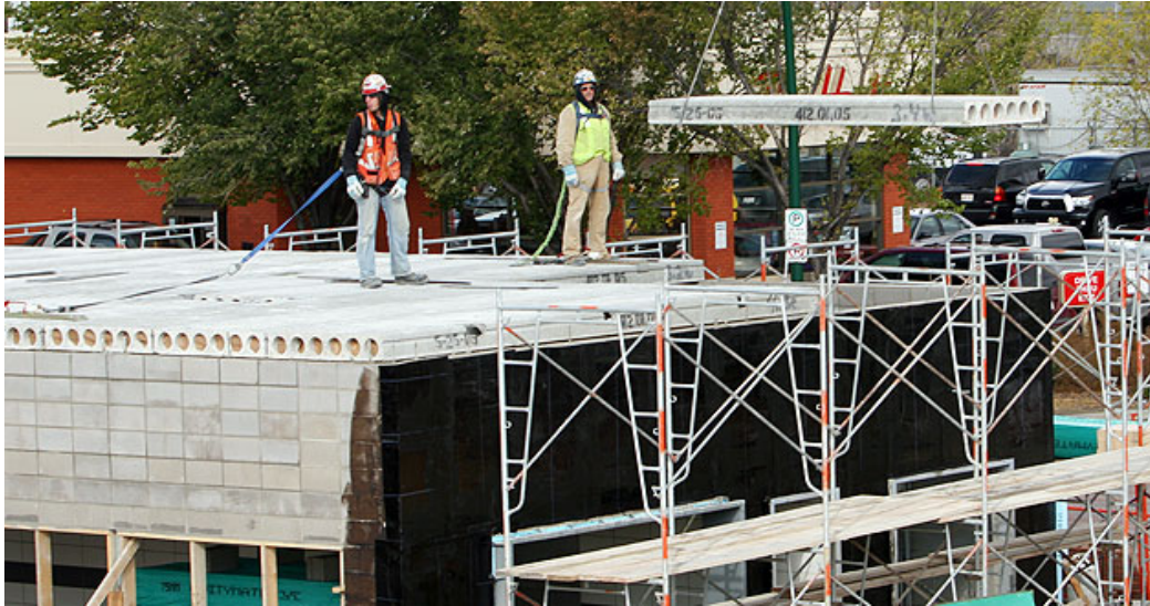
Pre-stressed hollow-core slabs are cast according to Customer dimensions
